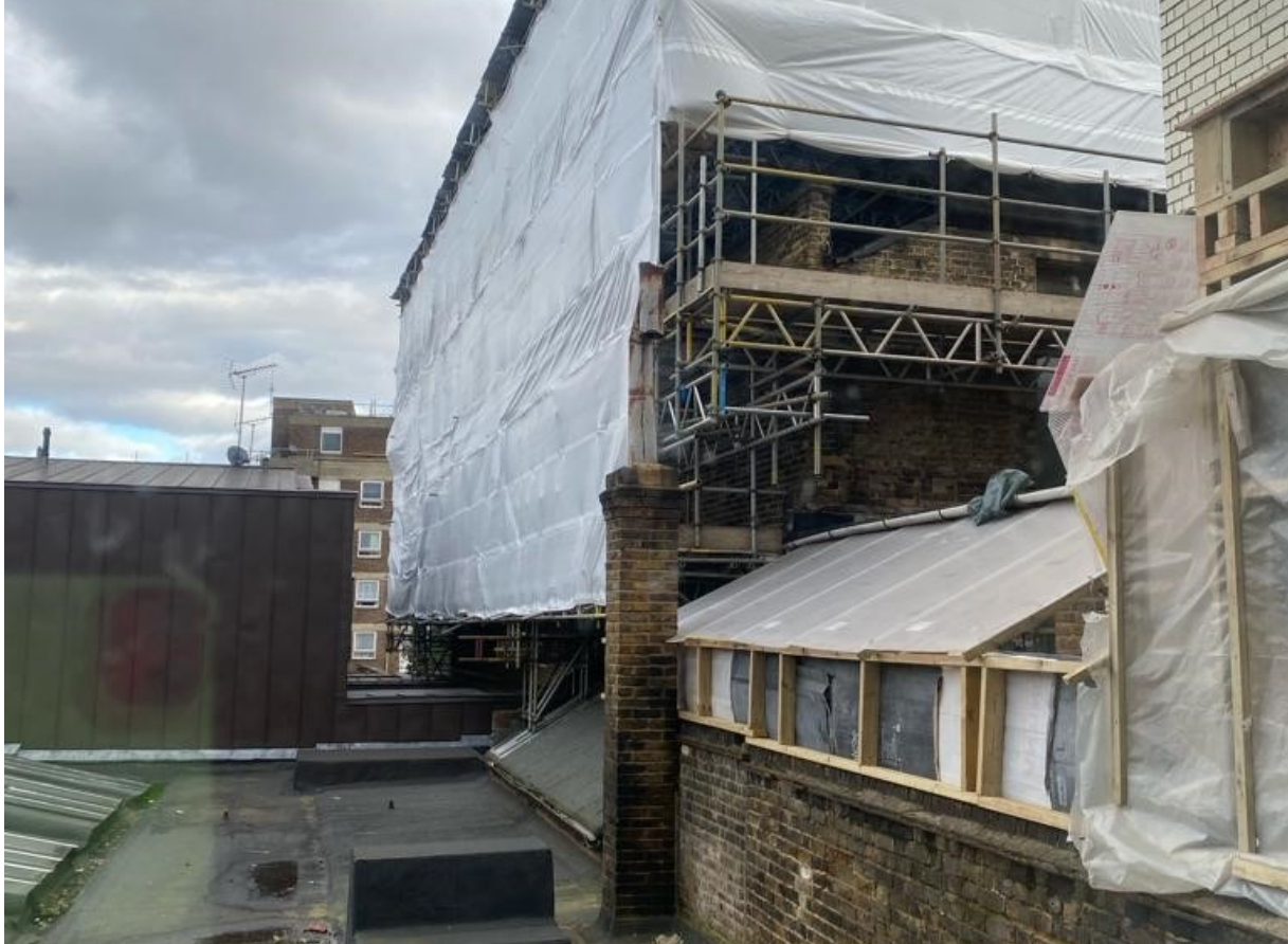
WORKS IN PROGRESS TO THE LARGE HALL ROOF
